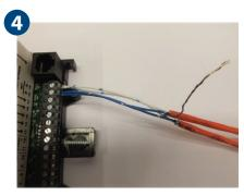
Twist shield wires together to form good electrical connection.
